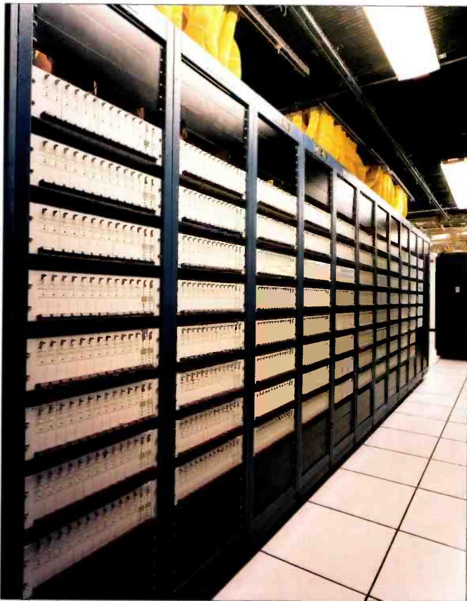
The facility's routing system employs 1024 Grass Valley Group 1x9 digital DAs feeding 32 routing frames.
