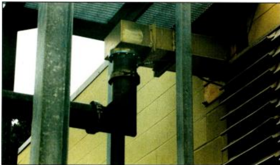
Tuning is important in systems used for multiple channels. Placing elbows too close to each other can increase the complexity of tuning the system.
